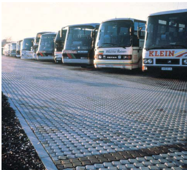
Extensive areas of concrete block permeable paving for bus parking areas at the World Exposition, Hanover, in 2000.
