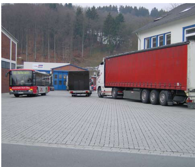
Permeable paving used for heavily trafficked industrial areas in Germany
